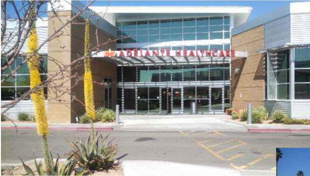
Main Entry to Adelante Healthcare Facility in Mesa
