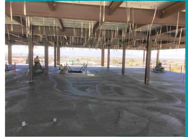
Level 5 Concrete Finishing
