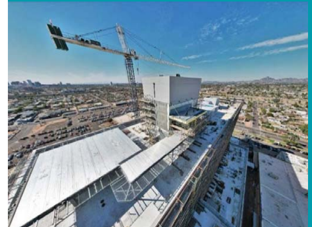
Helipad and Catwalk Progress
