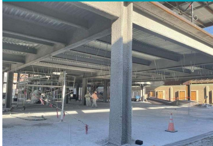
Level 1, Soundcrete Monocote Detailing
