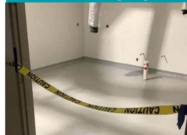
Basement Flooring Progress
