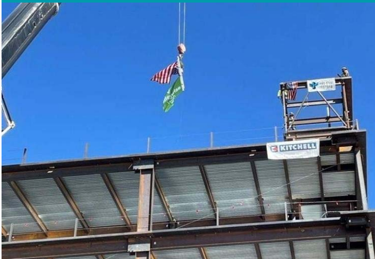
Topping Out Beam Being Placed
