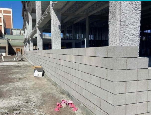
CMU Block Wall Progress
