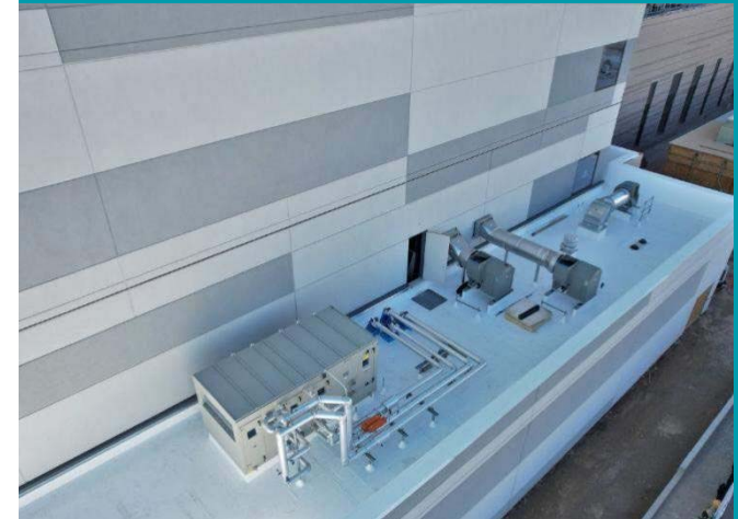
Roof 1 Mech. Equipment Install
