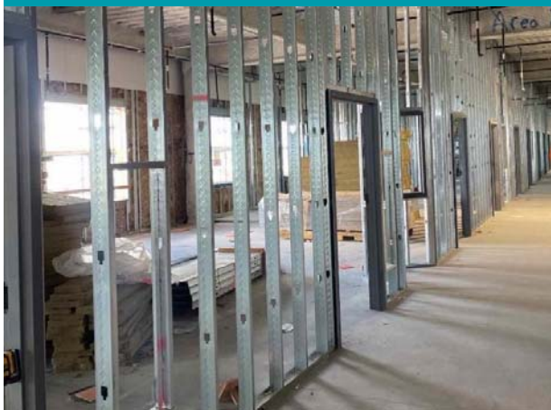
Floor 9 Framing Progress
