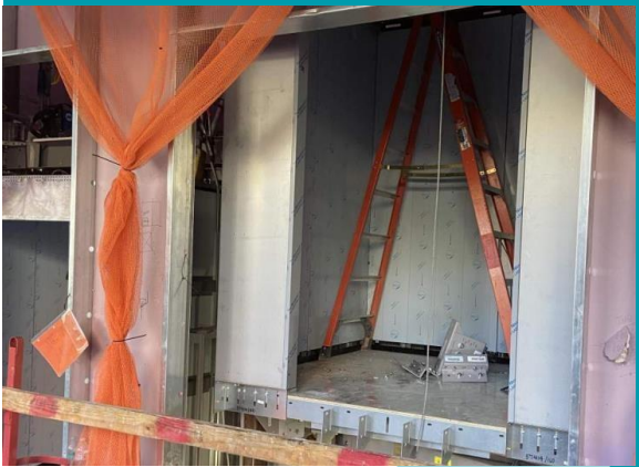
Elevator Cabs Build Out Underway
