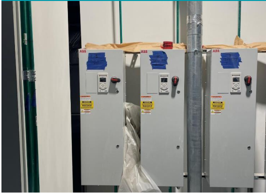
Level 3, Pneumatic Tube Install
