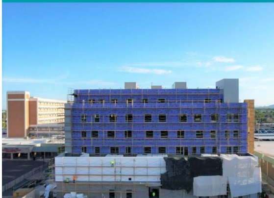
Drone Photo- South Elevation
