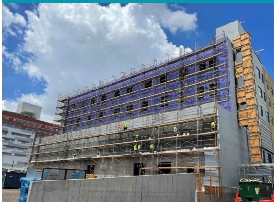
EIFS Brown Coat- South Elevation
