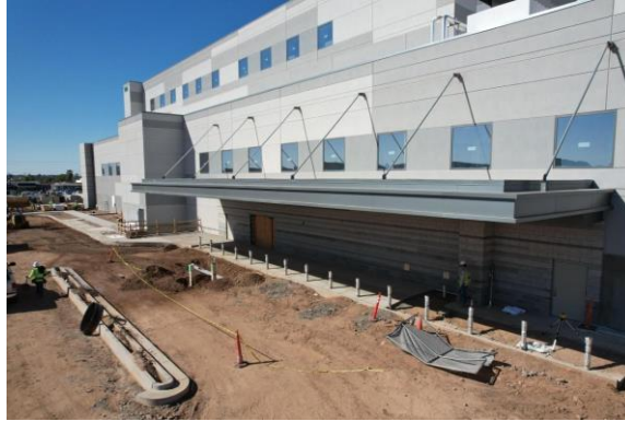
Phase 1, Curb / Sidewalk Progress
