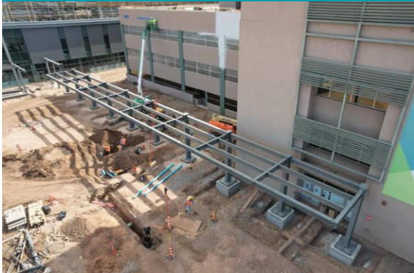
NW Canopy, Steel Progress
