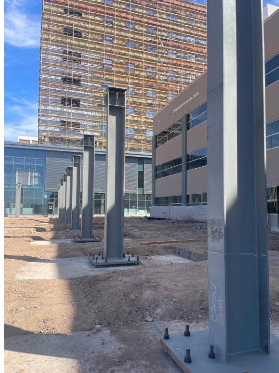
Northwest Canopy Steel Install
