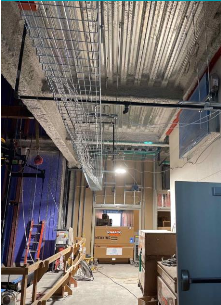
Level 1, Cable Tray Install
