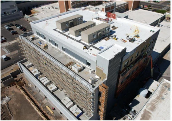
South and East Elevations
