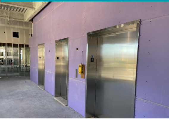
Elevator Front Buildout
