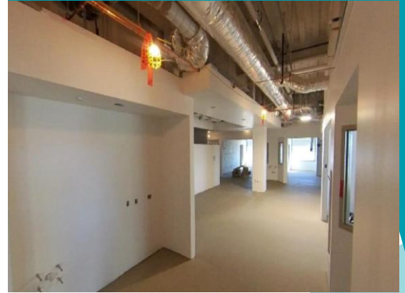
Level 6, Paint Progress
