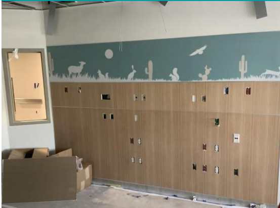
Level 4, Headwall Finishes
