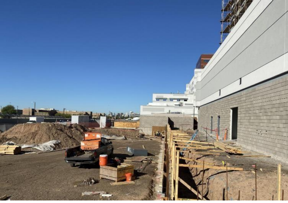
Loading Dock Footings
