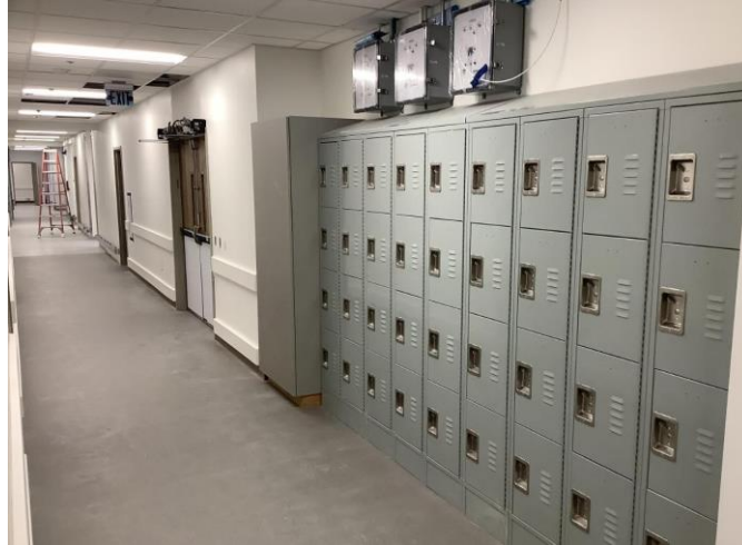
Basement Locker Installation
