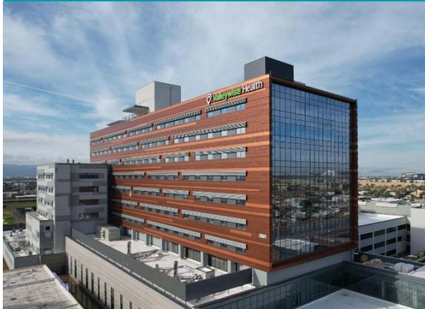
Exterior Signage East Side
