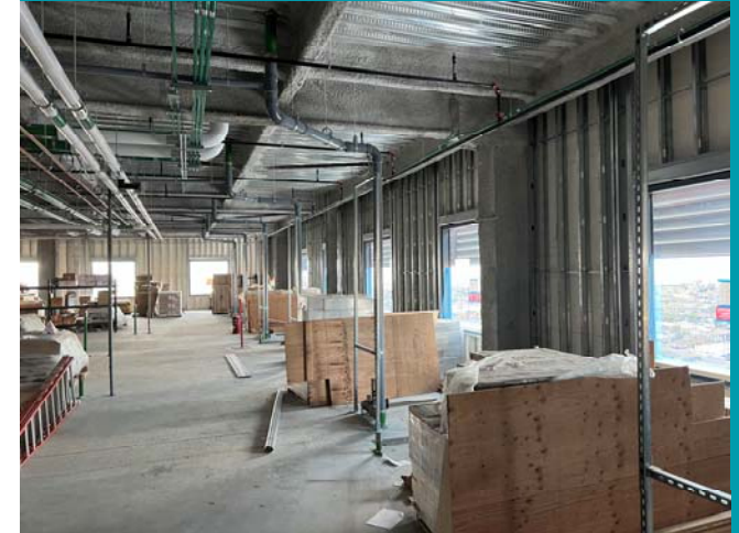
10 th Level, Plumbing Rough-In
