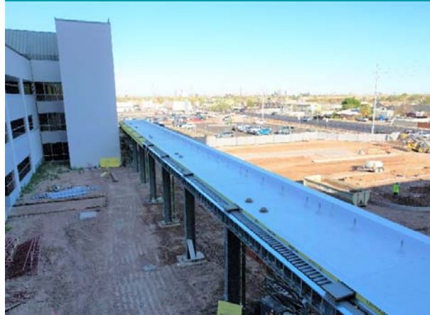
North Canopy Progress
