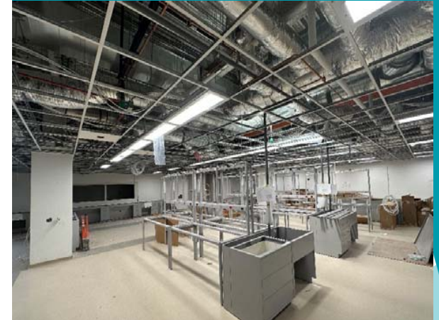
Level 3, Lab Progress
