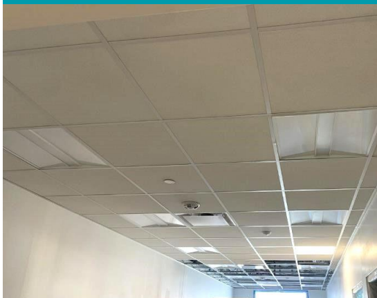
Level 5, Ceiling Tile Install
