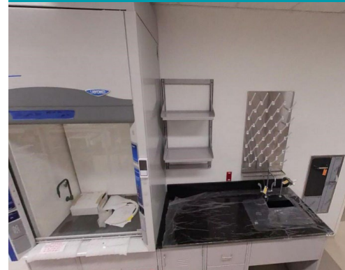
Level 3, Lab Progress
